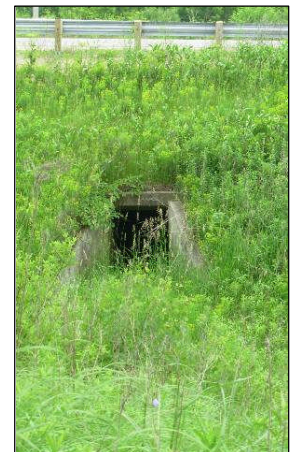
The cow tunnel could provide access under USH 14 if reconfigured.
