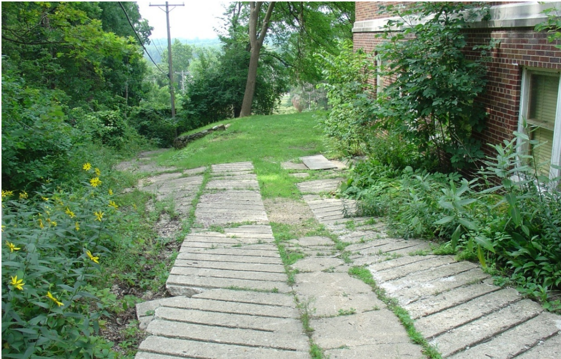
Figure 3- 33: Remnants of concrete service driveway at east side of Dormitory, 2010. 6215
