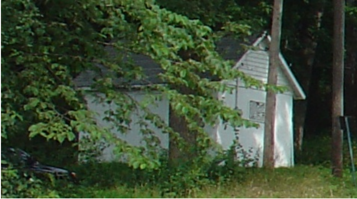
Figure 3- 6: Old Water Utility Building, south and east elevations, 2010. (source: QEA 3161).
