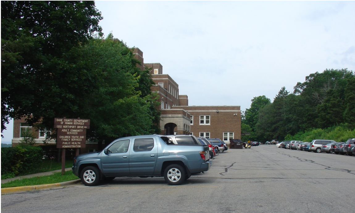
Figure 3- 38: Parking lot at north side of building, facing west, 2010. (source: QEA 6026)
