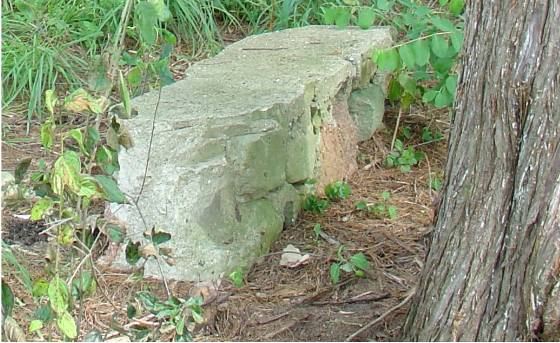
Figure 3- 26: Remnants of stone bench near retaining wall, 2010 (source: QEA 6292)
