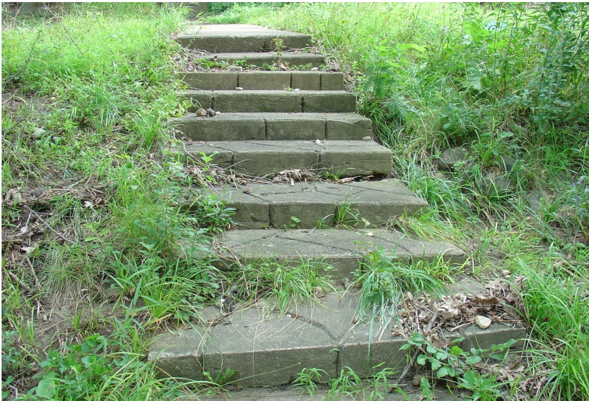
Figure 3- 29: Stamped concrete steps, 2010. (source: QEA 6320)
