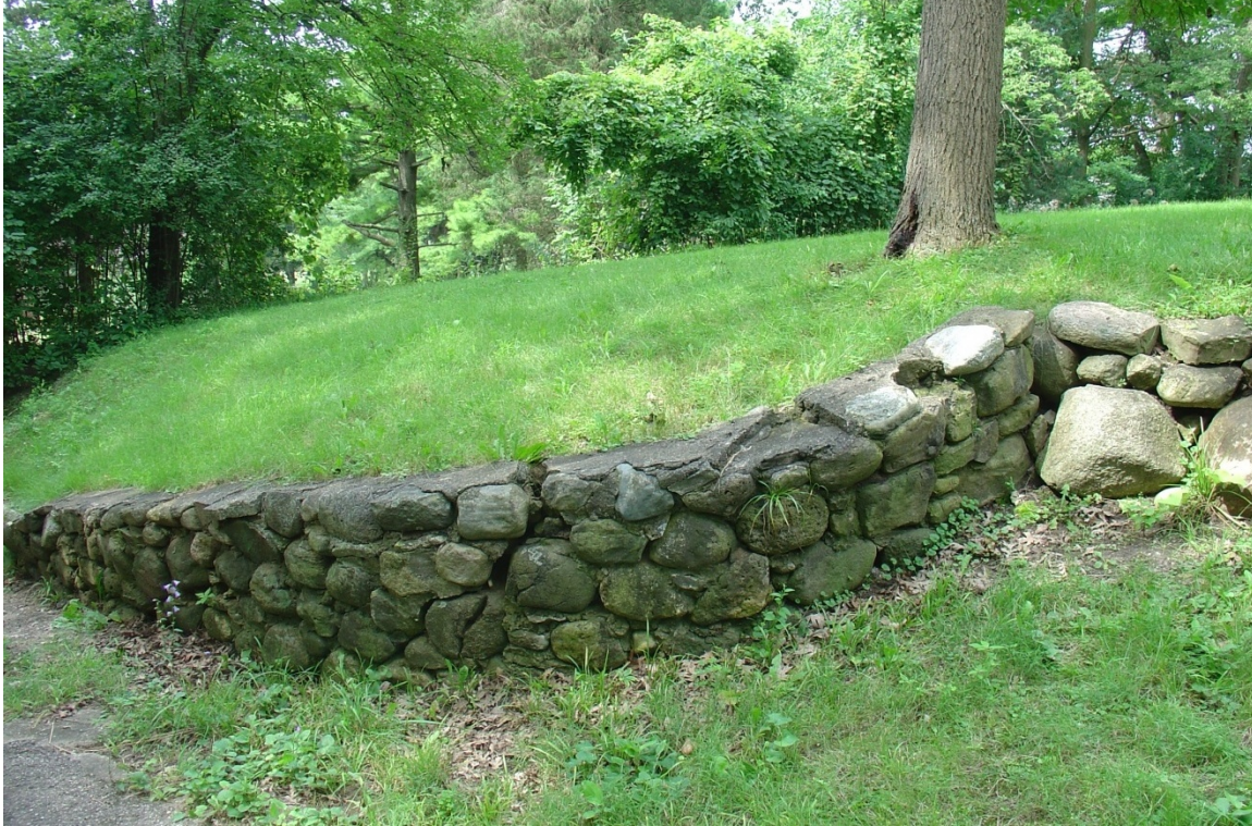
Figure 3- 36: Remnants of stone retaining wall near Dormitory, 2010 (source: QEA 6250)
