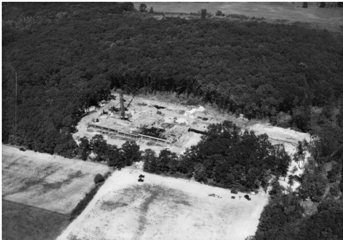
Figure 2- 4: Lake View Sanatorium under construction, 1929. (source: Wisconsin State Historical Society Archives, 35103, by Athur M. Vinje).
