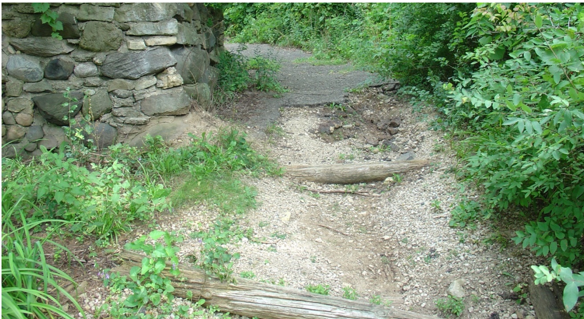
Figure 3- 35: Erosion at former service road, 2010 (source: QEA 6266)
