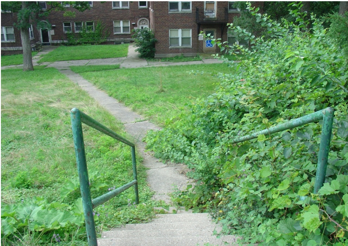
Figure 3- 27: Concrete steps between parking lot and Dormitory, 2010. (source: QEA 6040)
