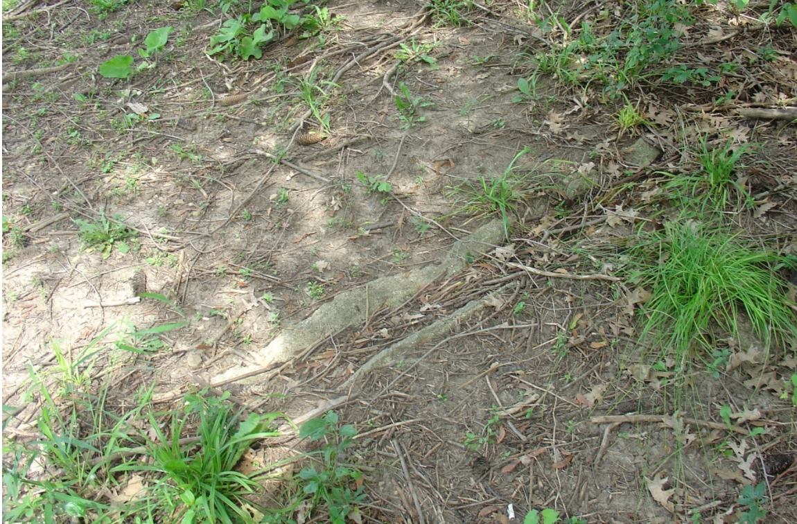
Figure 3- 18: Remnant of cement drainage channel at western side of Dormitory, 2010. (source: QEA 6342)
