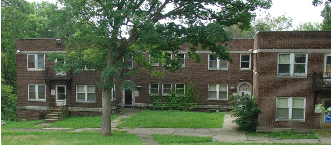
Figure 3- 12: Dormitory for Help, portion of the north elevation, 2010. (source: QEA, 6042)
