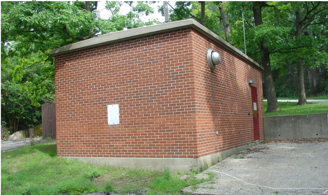
Figure 3- 11: Pump House, 2010. (source: QEA 6187)
