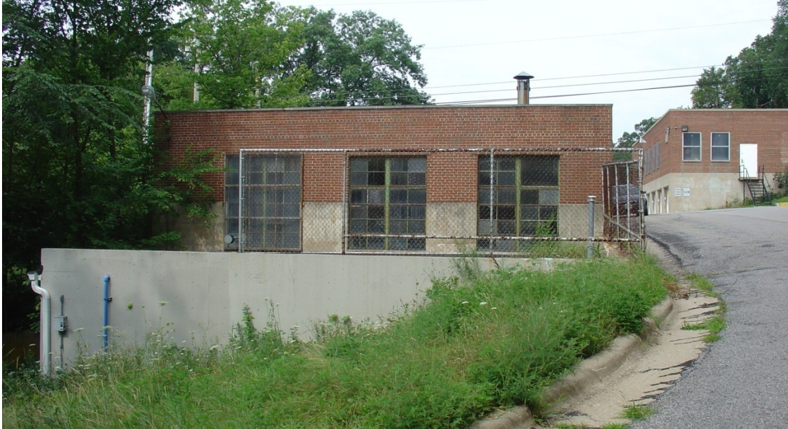
Figure 3- 10: Power House, East Elevation, 2010. Note: the garage is in the background on the right of the image. (source: QEA 6154)
