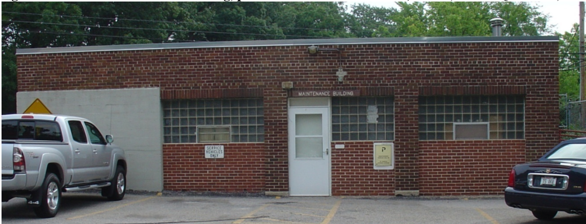
Figure 3- 9: Maintenance Building, west elevation, 2010. (source: QEA 6036)
