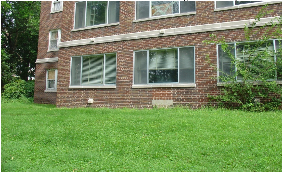
Figure 3- 31: Location of former southern door at Dormitory, 2010. (source: QEA 6338)
