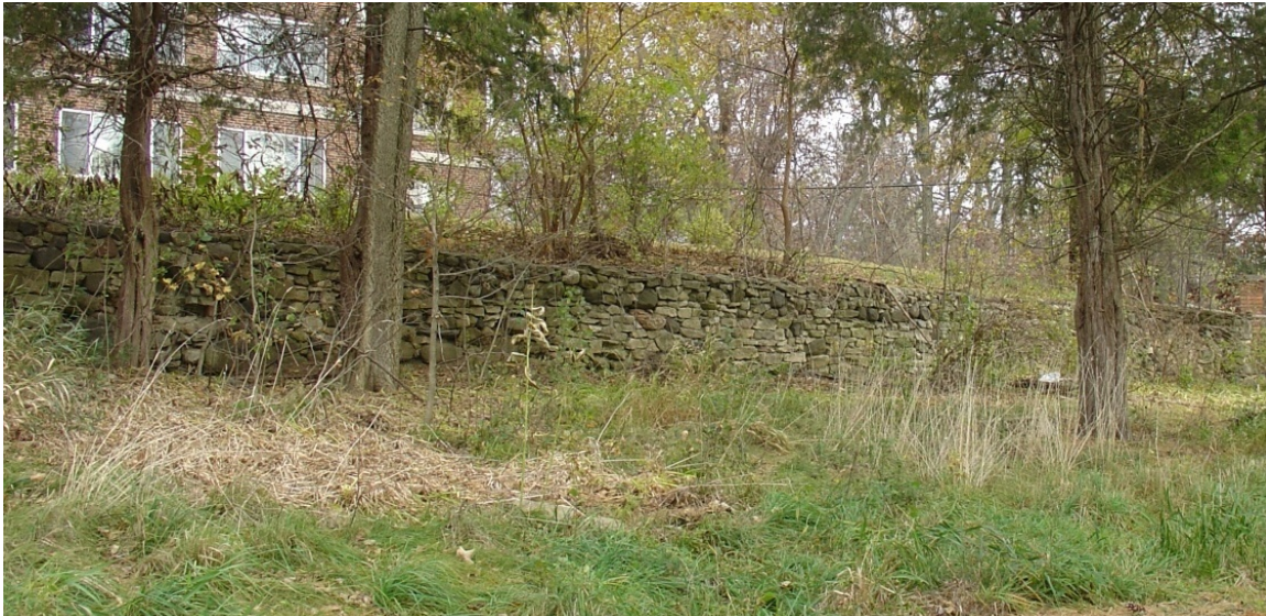
Figure 3- 23: Rubble stone retaining wall south of Dormitory for Help, 2010. (source: QEA 7600)
