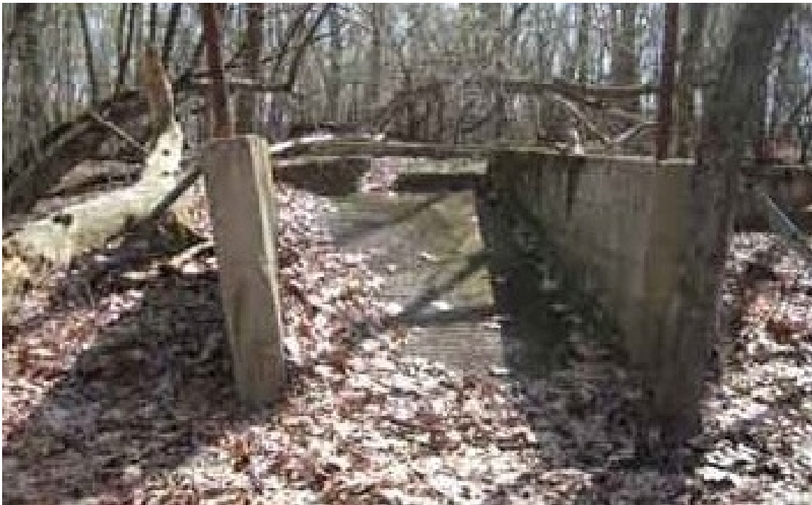
Figure 3- 57: Foundation of Hog Barn, 2008 (source: Lake View Hill Master Plan)
