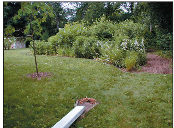
Figure 9: Downspout directed toward a rain garden. Source UW Extension.
