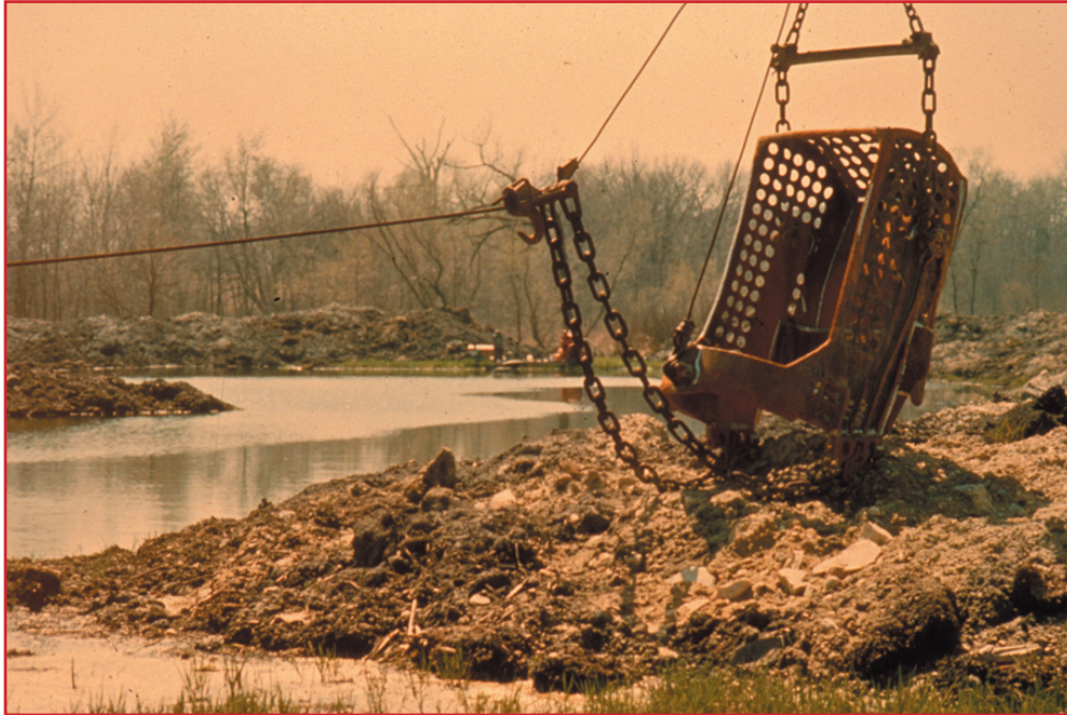
Figure 8: Dredging sediment from clogging a river. Source Wisconsin DNR.
