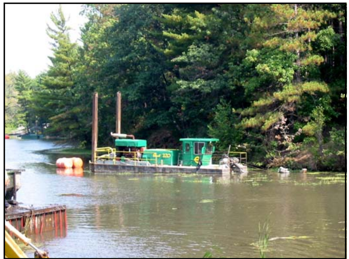
Hydraulic Dredging of Stewart Lake
