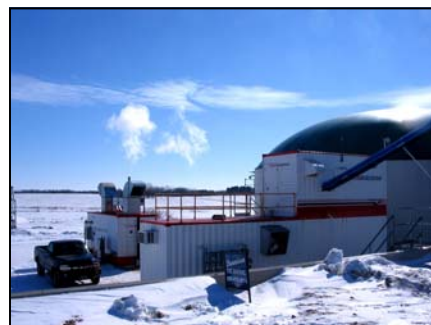
Manure digester on the Crave Brothers Farm
