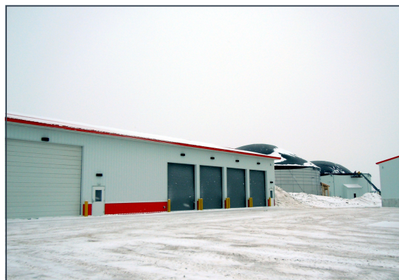
Solids storage building and digester tanks
