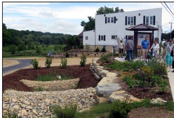
Completed Rockdale Mill Site
