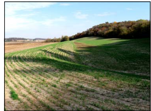
Grade Stabilization Structure: This structure effectively traps suspended sediments and corresponding particulate phosphorus, preventing it from reaching nearby surface waters.
