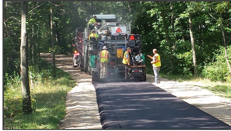
Phase 1 Lower Yahara River Trail Construction
