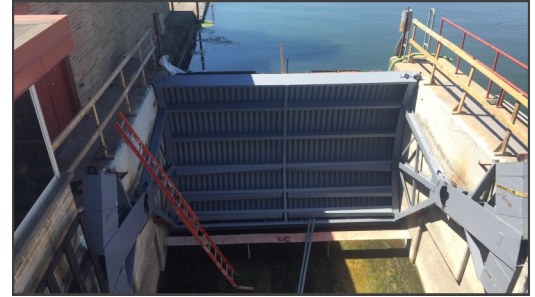
Above: Old lock gate Below: Newly-installed lock gate
