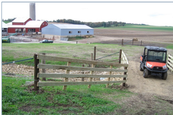
Photo of a stream crossing and rock lined waterway
