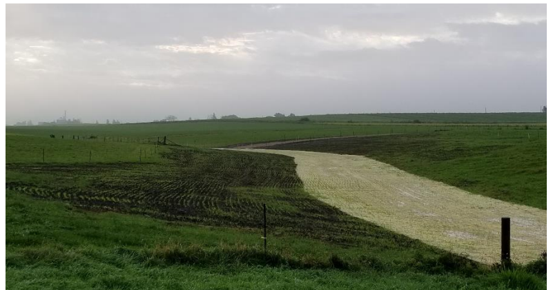
Participants registering for the Dane County Grazing Workshop (top photo). Grassed waterway installed to address gully erosion (bottom photo).
