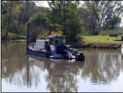
Hydraulic dredge removing legacy sediments from Token Creek.
